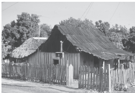
FIGURE 5. REDESIGN —a tandem plan construction with a Type 3 structure in front and a Type 1 structure at the back.
